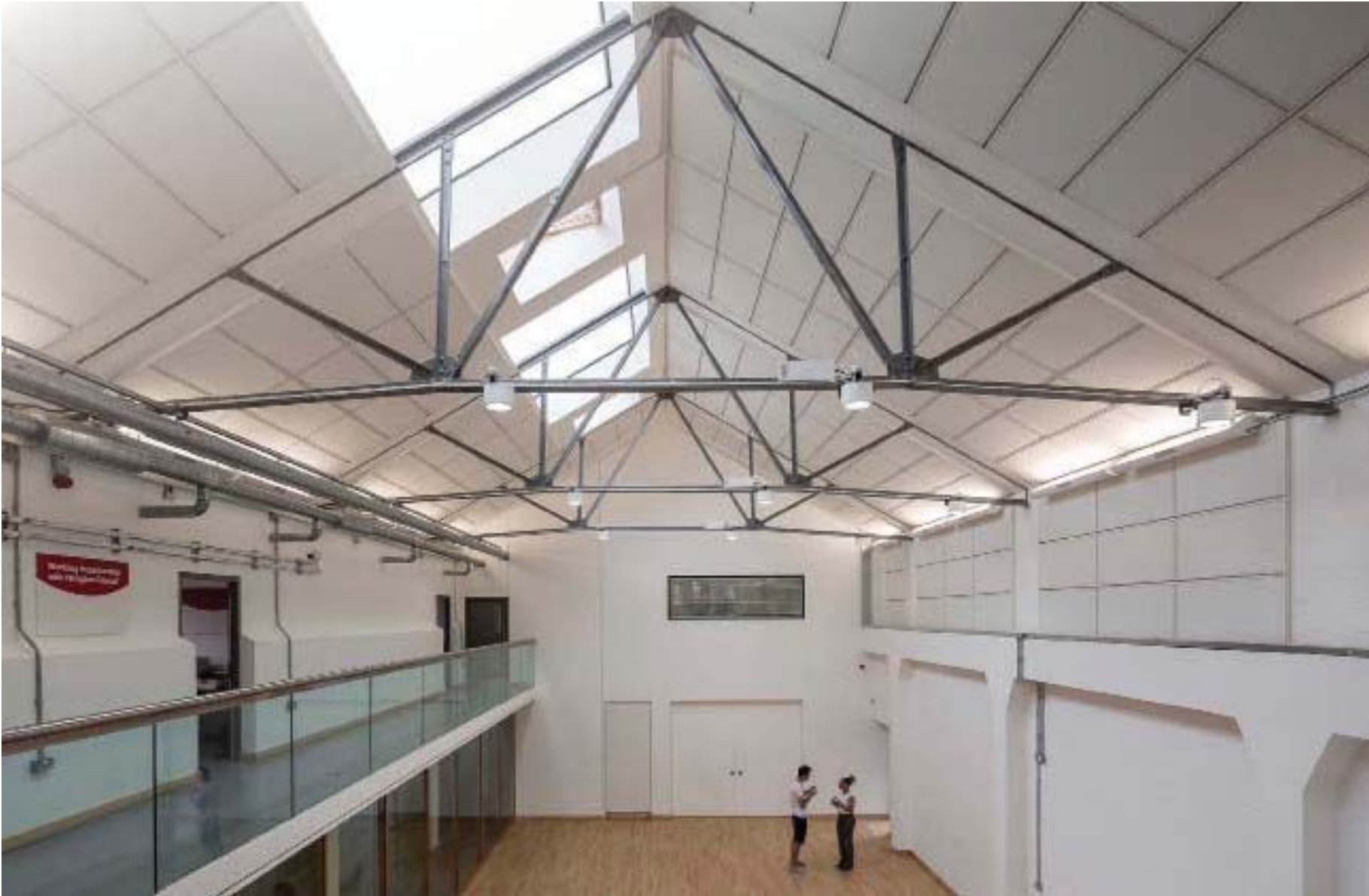
The main hall after refurbishment
