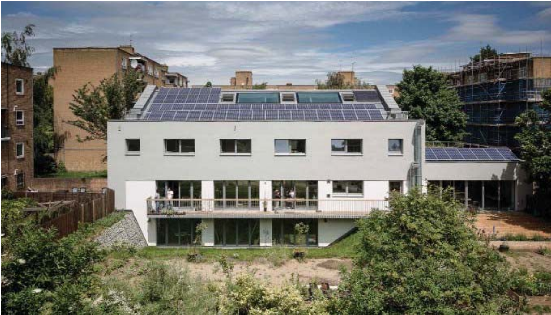
The refurbished Mayville Community Centre South Facade
