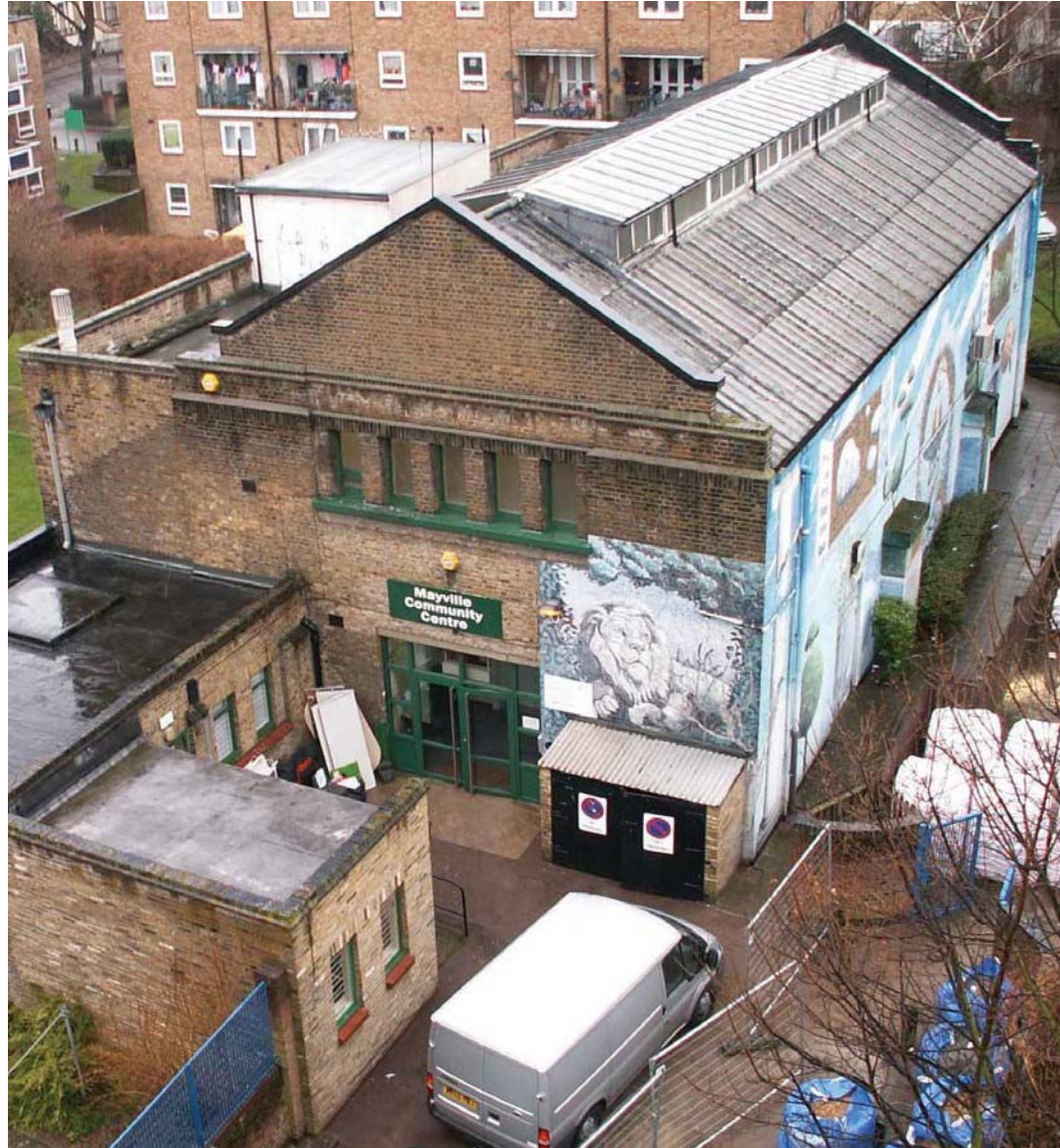
South elevation before refurbishment
