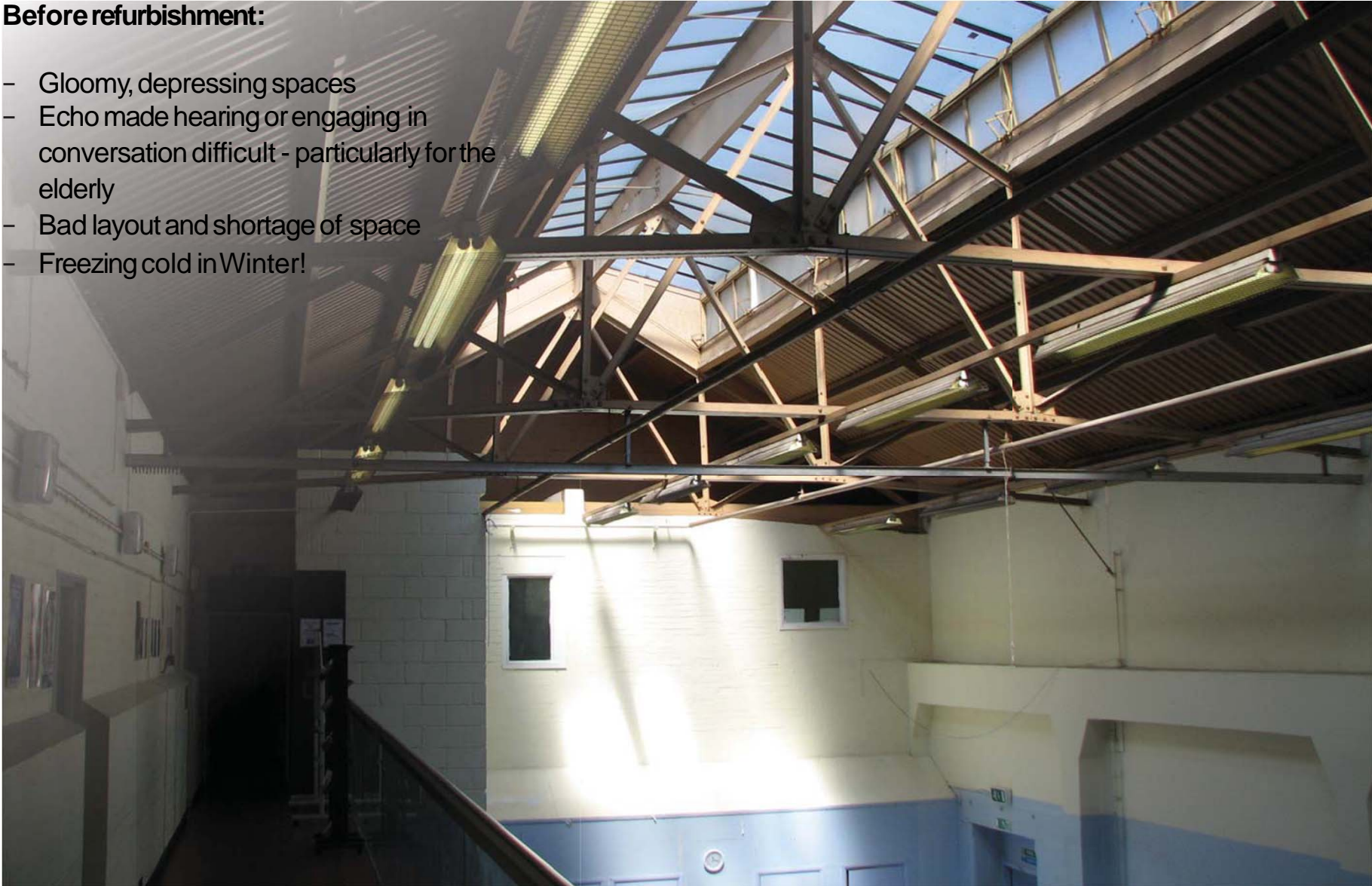
The main hall before refurbishment
