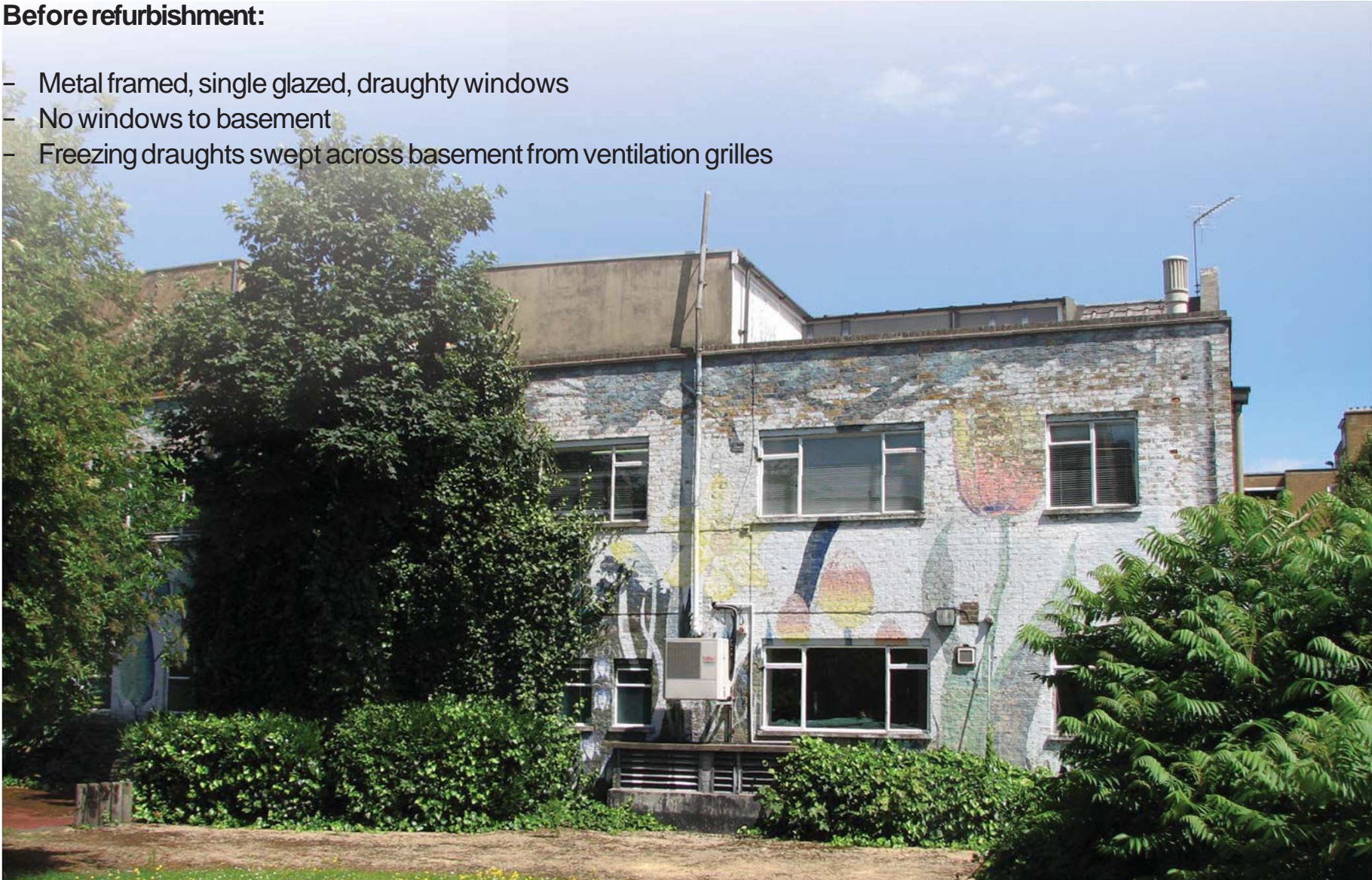
South elevation before refurbishment
