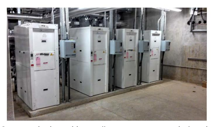
2-stage design with scroll compressors and plate heat exchangers. Any HP can be used for heating or cooling
