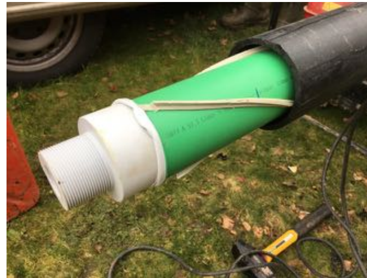
On-site prototype assembly
