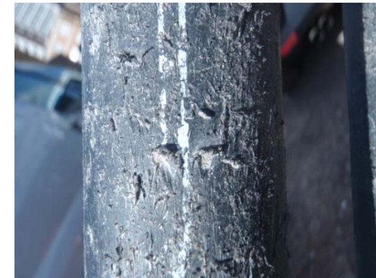
Lower pipe after test
