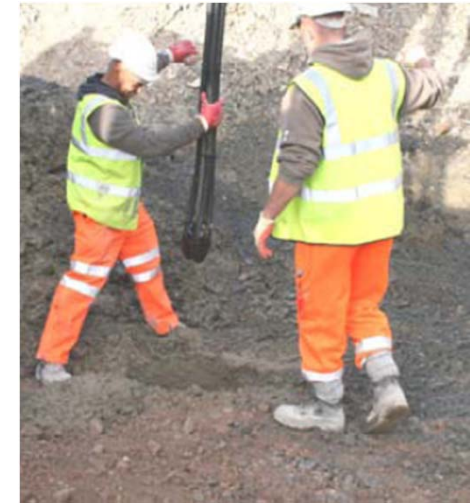
Plunging used T32 bar + 4 pipes (2 loops)
