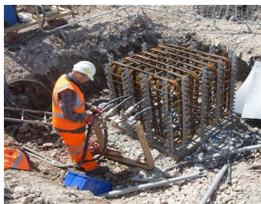
Energy Pile Installation
