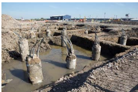
Energy Pile Installation
