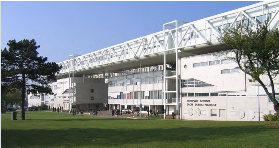
Left: University of Burgundy. Source: University of Burgundy Right: The heat pump. Source: Tenova
